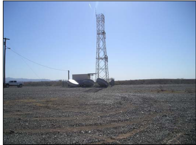
Photograph 4: View toward Vidal Junction candidate location, facing east.
